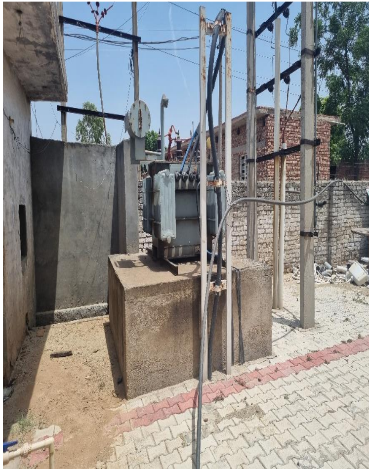
Figure 4.10 400KVA Transformer
