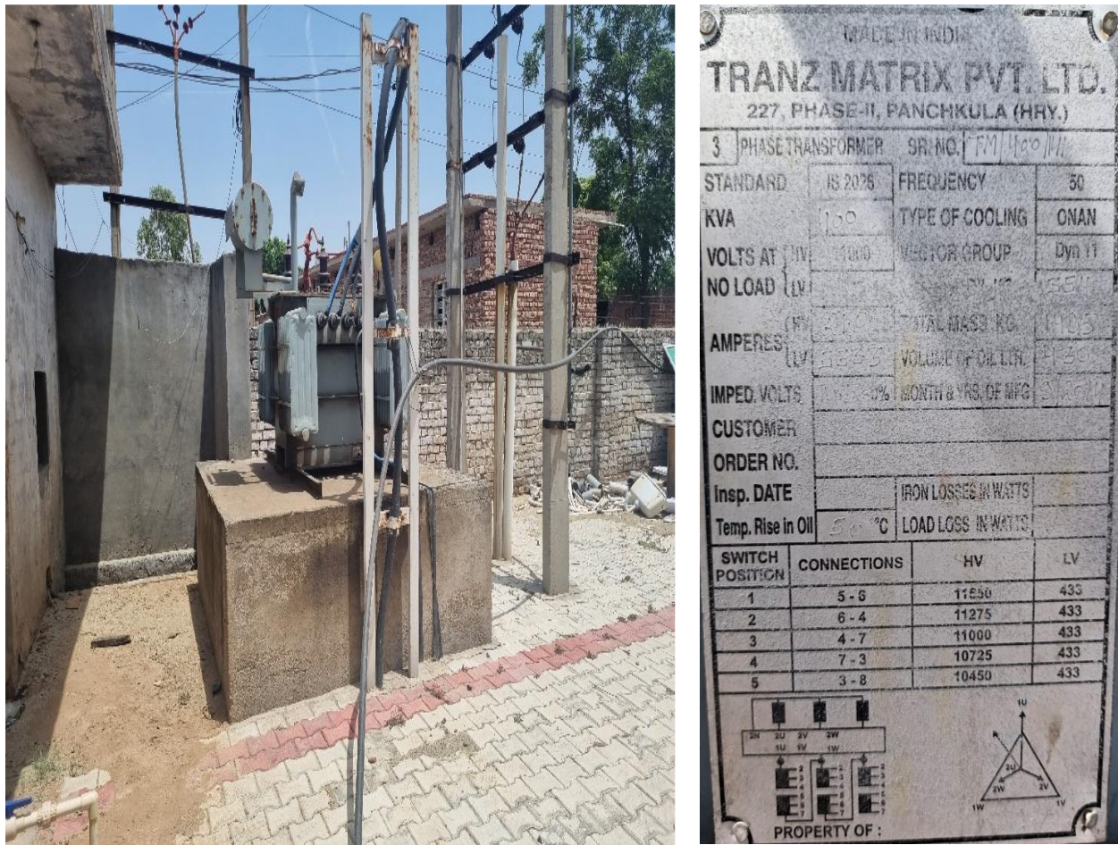
Figure 4-8 400KVA Transformer
