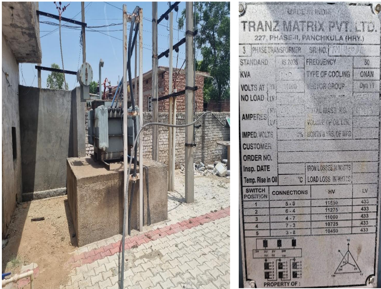
Figure 4-9 400KVA Transformer
